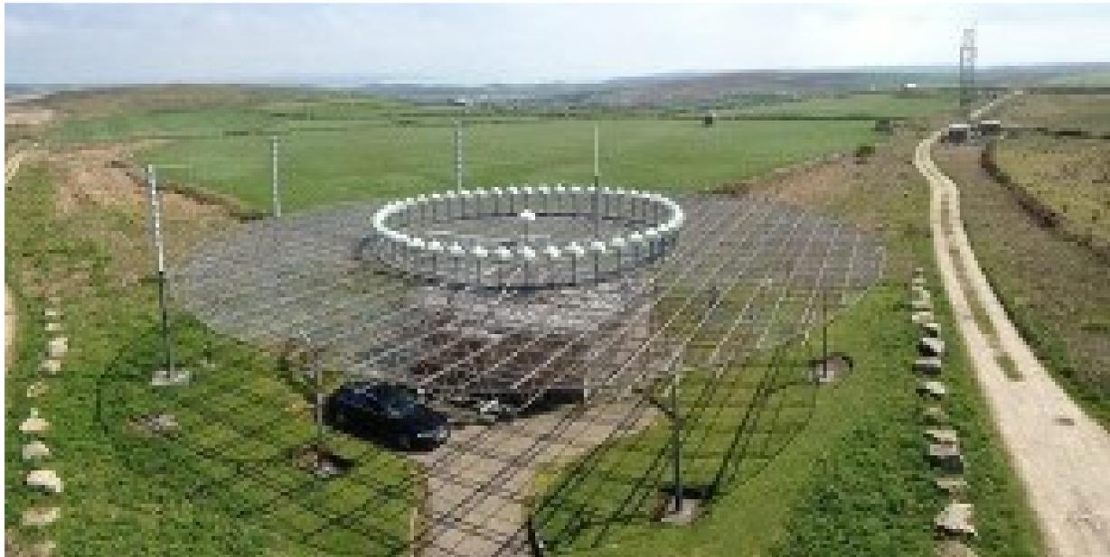
A VHF Omni direction Radio range (VOR) beacon with a car for scale (Image courtesy nats.aero)
